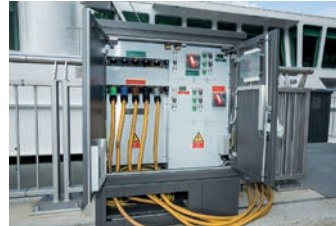
Power feeds for moored river and canal boats
