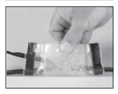
**3.6 Seal Film.** Seal film together between spacer pad and mastic.
